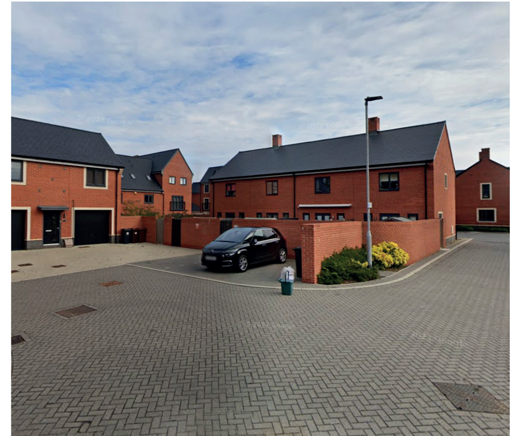
Fig.1 - Low density suburban development north of Colchester, where new homes are surrounded by hard standing to accommodate parked cars
