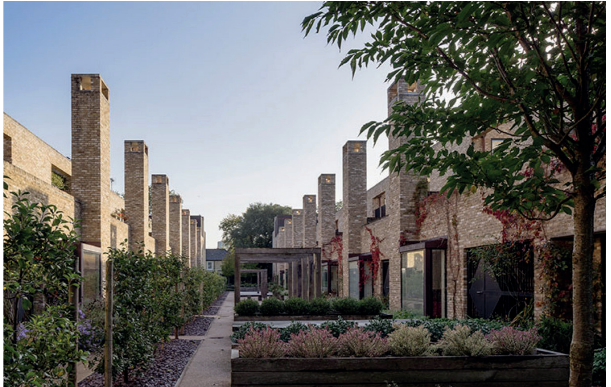
Fig. 124 - Accordia, in Cambridge. Is it possible to make this quality of housing development the standard across Essex, rather than the exception?
