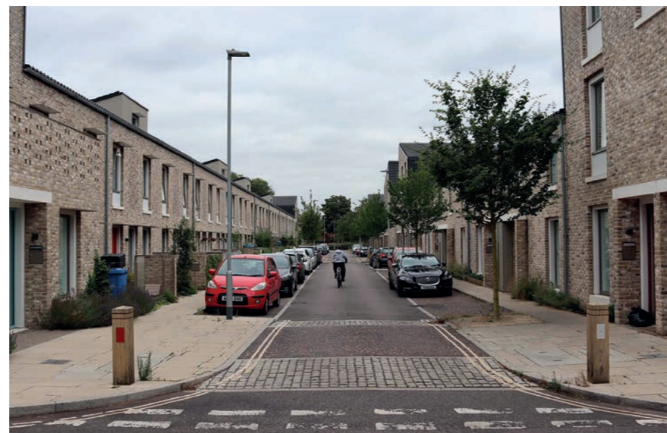
All car parking is accommodated on street at Goldsmith Street, which facilitates high density terraced housing with shallow back gardens
