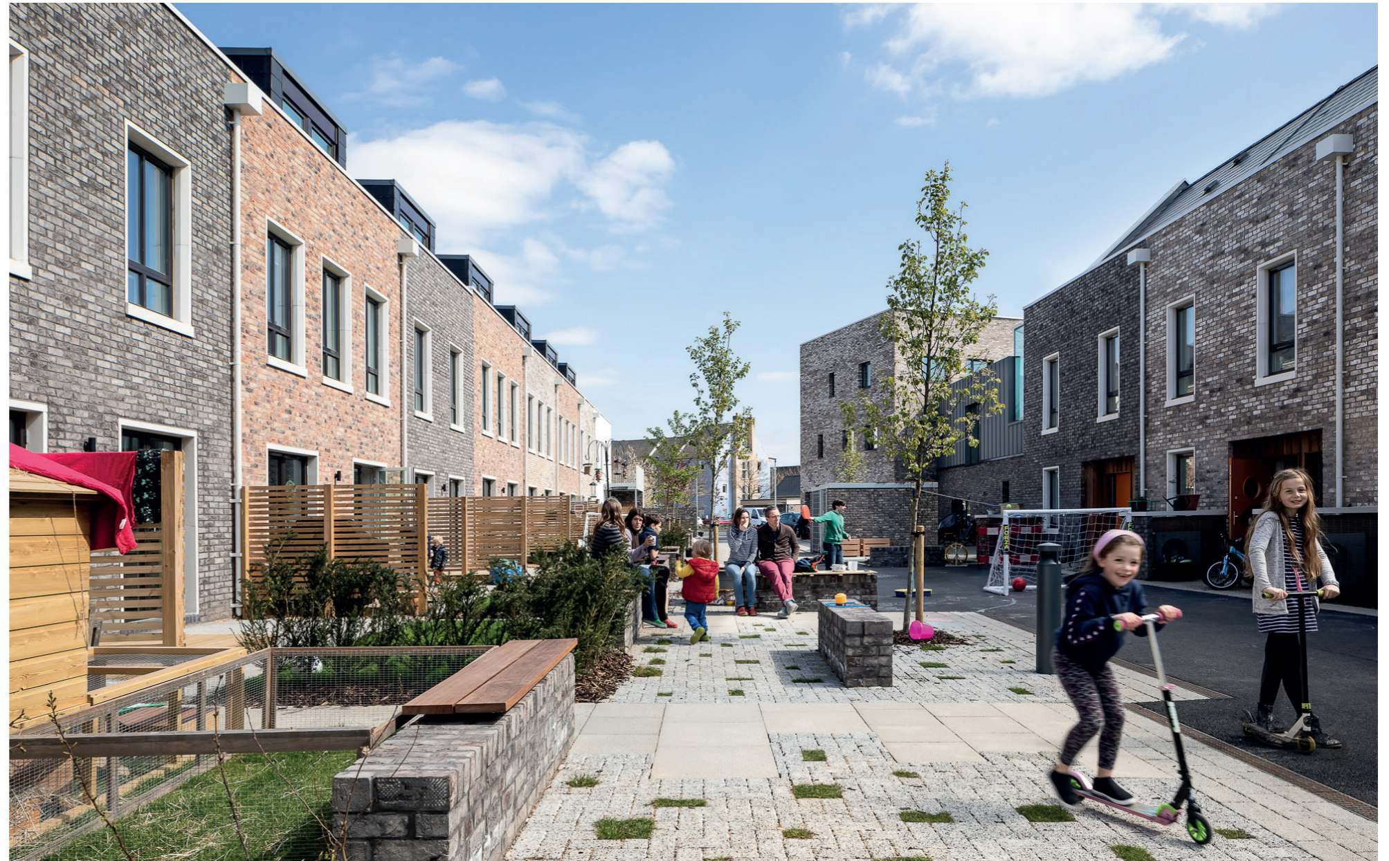
Fig. 159 - Marmalade Lane co-housing development.
