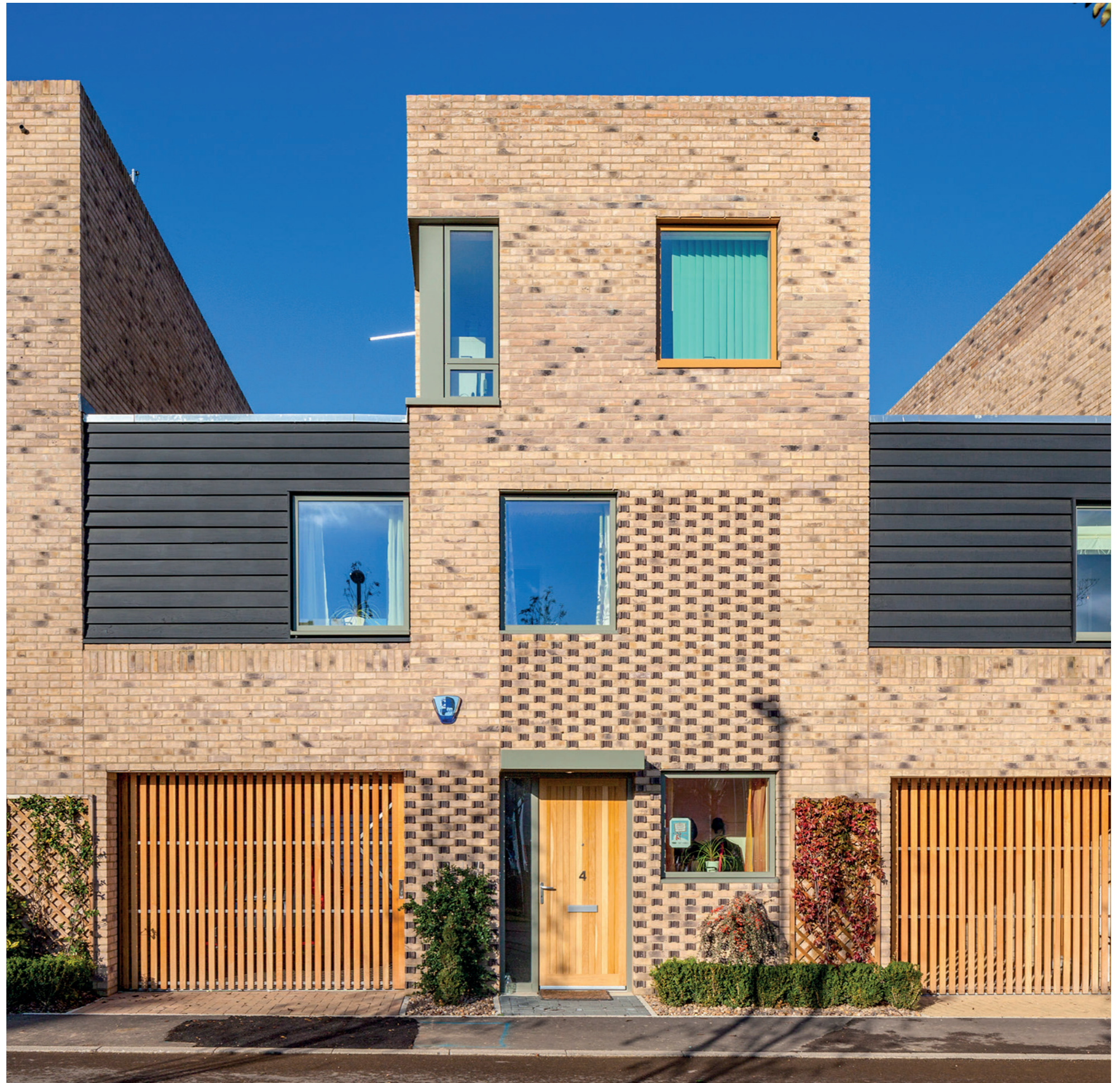
Fig. 53 Photograph of Abode, Great Kneighton (Image source: Proctor and Matthews Architects)
