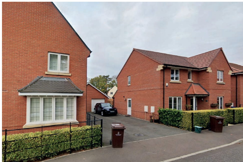
Figure 139 - The predilection of semi detached housing flanked by stacked parking limits densities and efficient form factors, as well as breaking up street frontage
