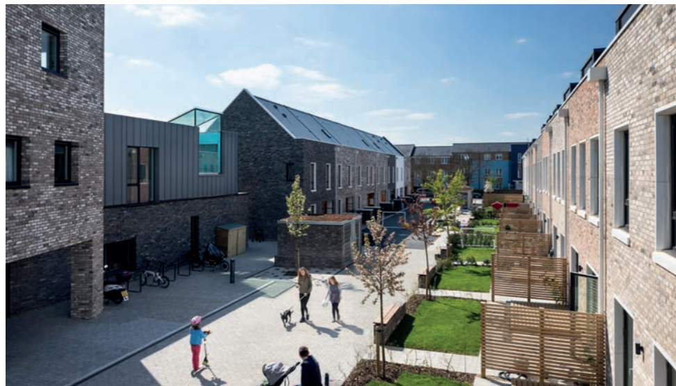
Fig. 158 - Marmalade Lane co-housing development
