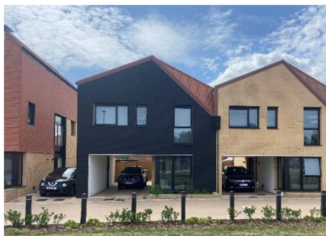
ITP – Fryerns (Basildon). Showing on plot parking incorporated into driveways and undercroft.
