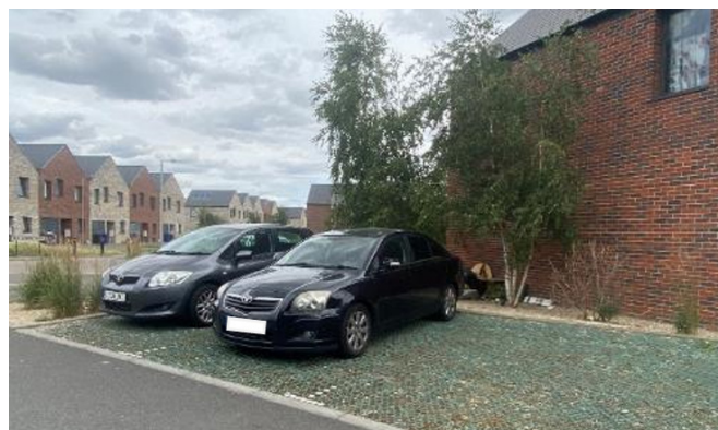
ITP – North View Avenue (Tilbury). Showing grasscrete parking areas, which can be more cost effective to remove compared with traditional surfaces (although maintenance implications of grasscrete should be considered).
